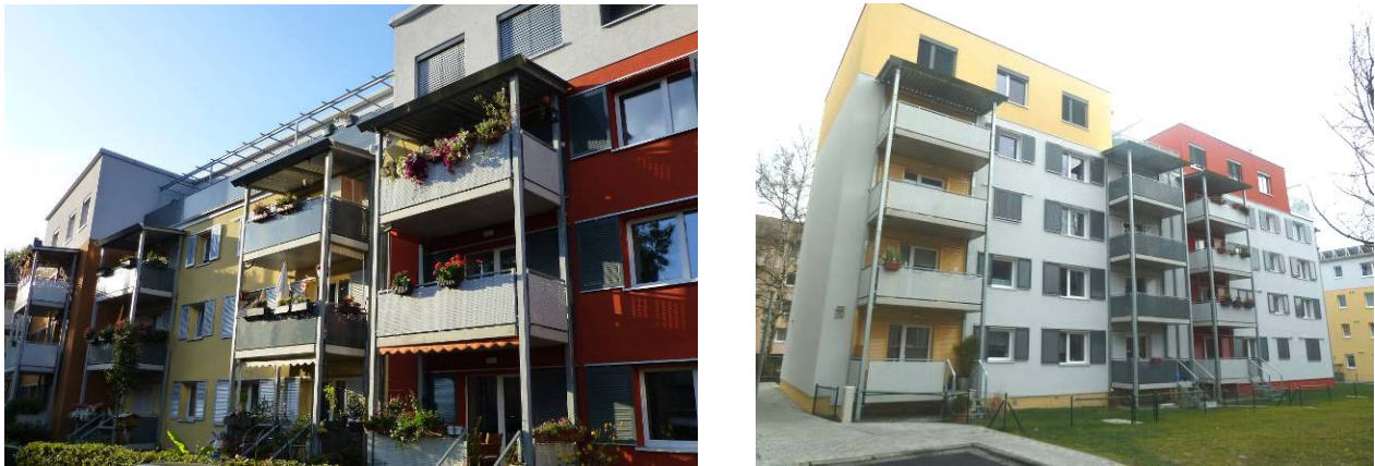
figure 1: External views of the buildings after retrofit
