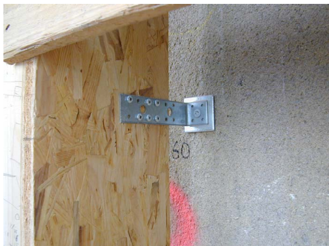
Image 1: Boxes of the façade insulation one storey in height (left), fastening of the profiles 5 cm in front of the existing wall by metal brackets for thermal isolation (right)
