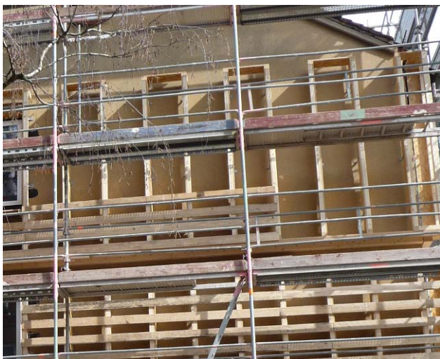
Image 1: Boxes of the façade insulation one storey in height (left), fastening of the profiles 5 cm in front of the existing wall by metal brackets for thermal isolation (right)
