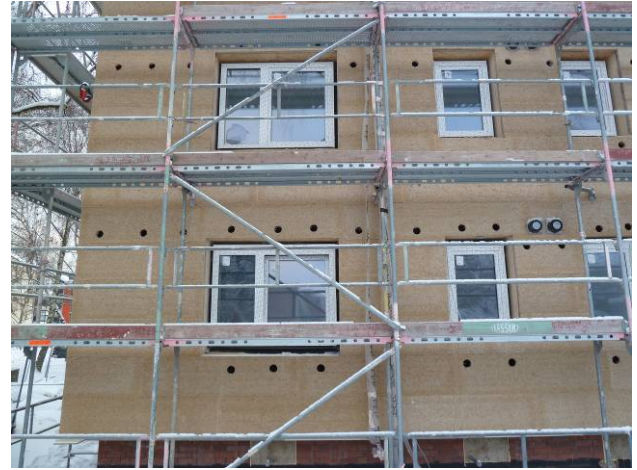
Image 2: Wooden planks on the substructure on a sample wall (left) as underground for wood wool panels with drilled holes to blow-in the cellulose in the hollow space (right)
