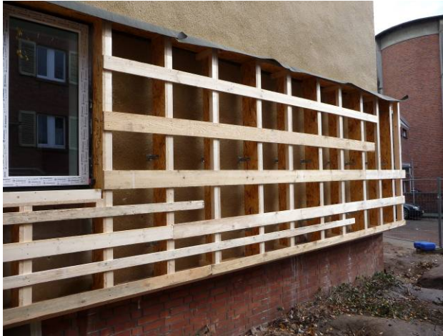
Image 2: Wooden planks on the substructure on a sample wall (left) as underground for wood wool panels with drilled holes to blow-in the cellulose in the hollow space (right)
