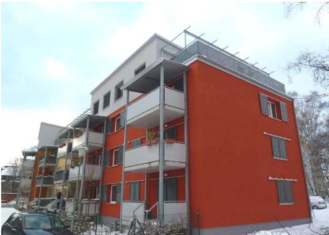
Image 6: The first construction phase
