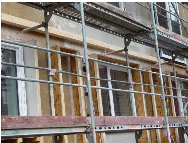
Image 3: Border strip of the windows with OSB-panels and gypsum fibre plates (left), insulation of the window frame with a mineral fibre plate (right)
