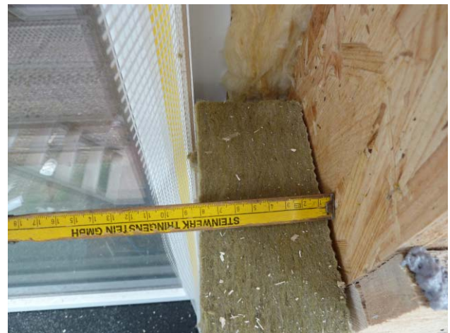
Image 3: Border strip of the windows with OSB-panels and gypsum fibre plates (left), insulation of the window frame with a mineral fibre plate (right)
