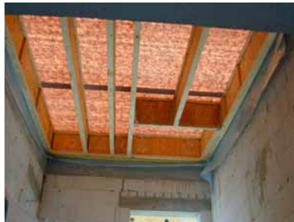
View on the light weight construction before closing and blowing-in the cellulose in the hollow space (40 cm)
