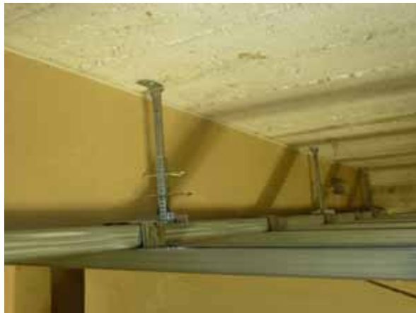
Mounting the suspension
