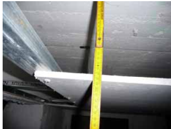
Hollow space of 26 cm for cellulose insulation
