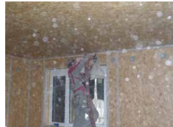
Filling the elements with cellulose
