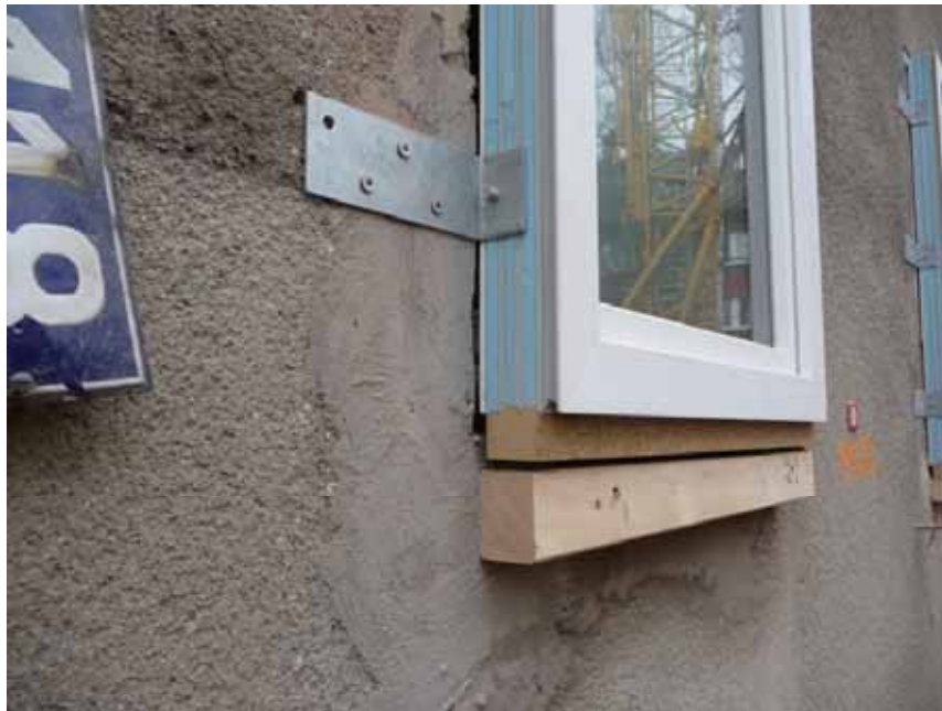
Mounting of the passive house windows in front of the existing walls with a thermal separation out of Purenit
