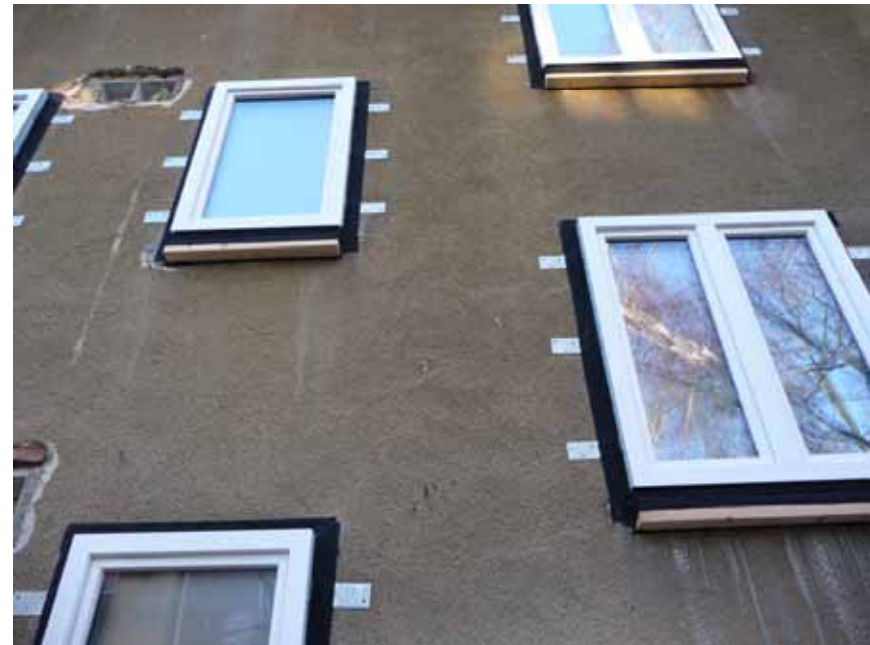
Sealing for airtightness on the existing outer plaster
