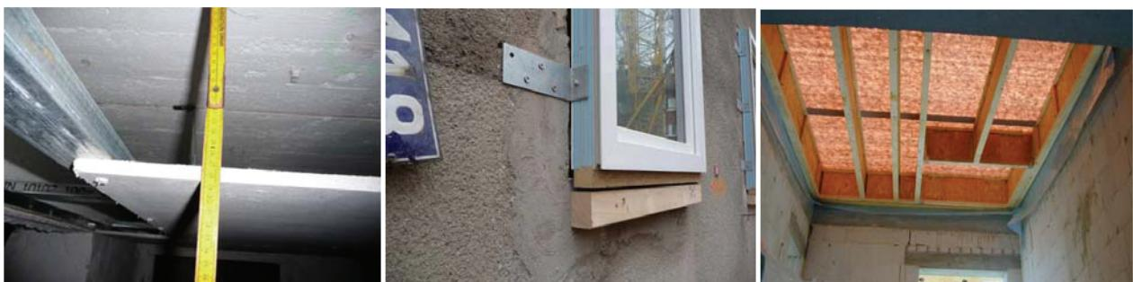
*Fig. 1: Hollow space of 26 cm for cellulose insulation in cellar (left), mounting of the passive house windows in front of existing wall (middle) and view of the light weight construction before closing and blowing-in the cellulose in the hollow space (40 cm)*
