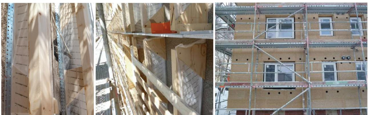
*Fig. 2: Details of the façade construction: thermally isolated sub construction with 29 cm thickness (left), horizontal separation between the floors with a fire protection panel, still without the mineral insulation plate (middle) and wood wool panels with drilled holes to blow-in the cellulose in the hollow space (right)*
