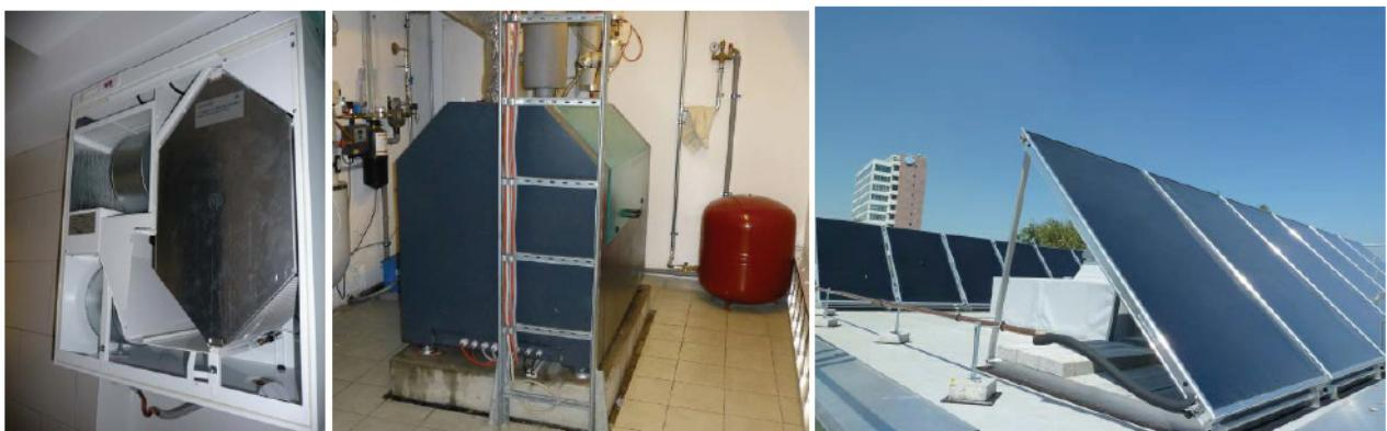
*Fig. 4: Mechanical ventilation in the bathroom of an apartment (left), rape-seed co-generation with 11 kW<sub>el</sub> and 22 kW<sub>th</sub> (middle) and thermal solar system on the roof during the mounting phase (right)*
